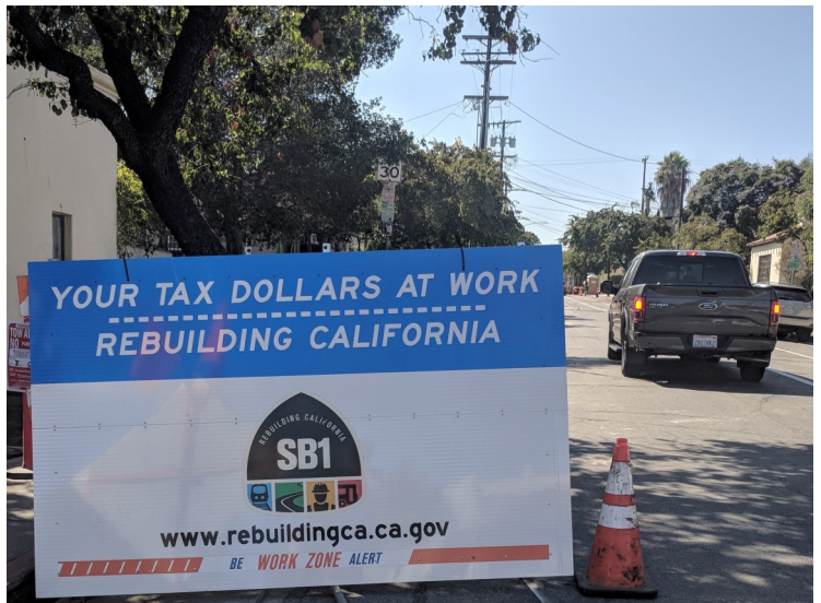
Road work on Bath Street
