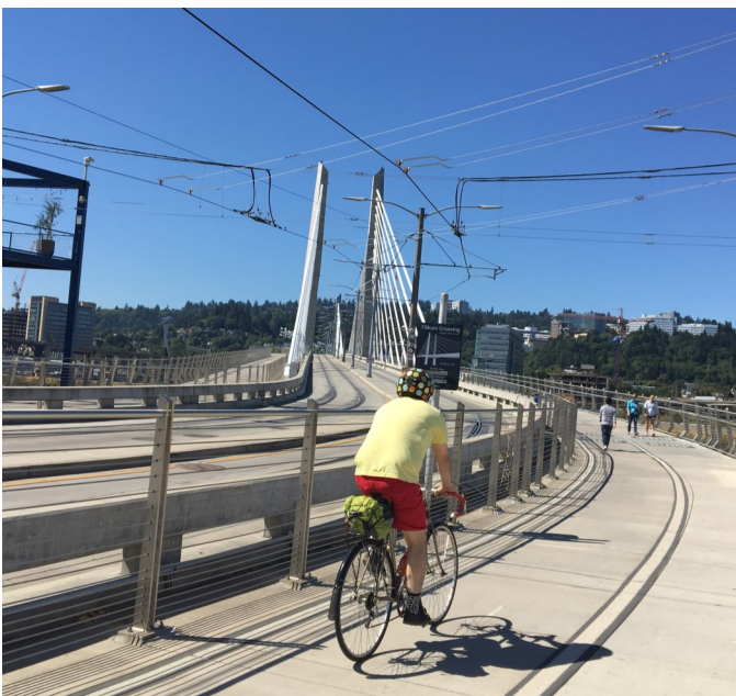
The Tilikum Crossing in Portland
